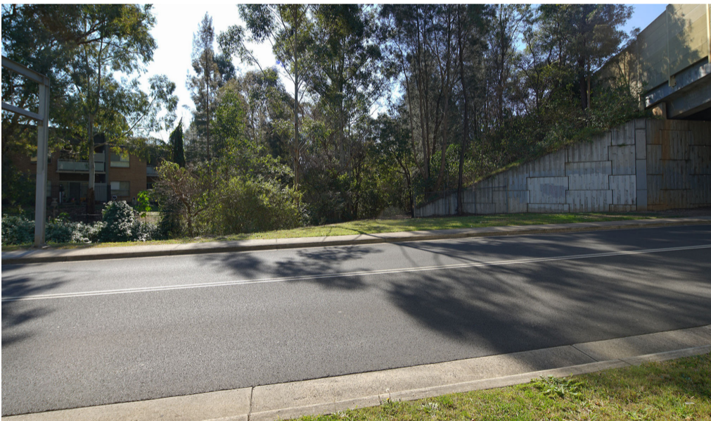
STREET VIEW LOOKING NORTH FROM PATTERSON STREET UNDERPASS
